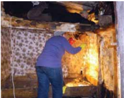
During treatment: passing the securing wire through the paper and ceiling boards
